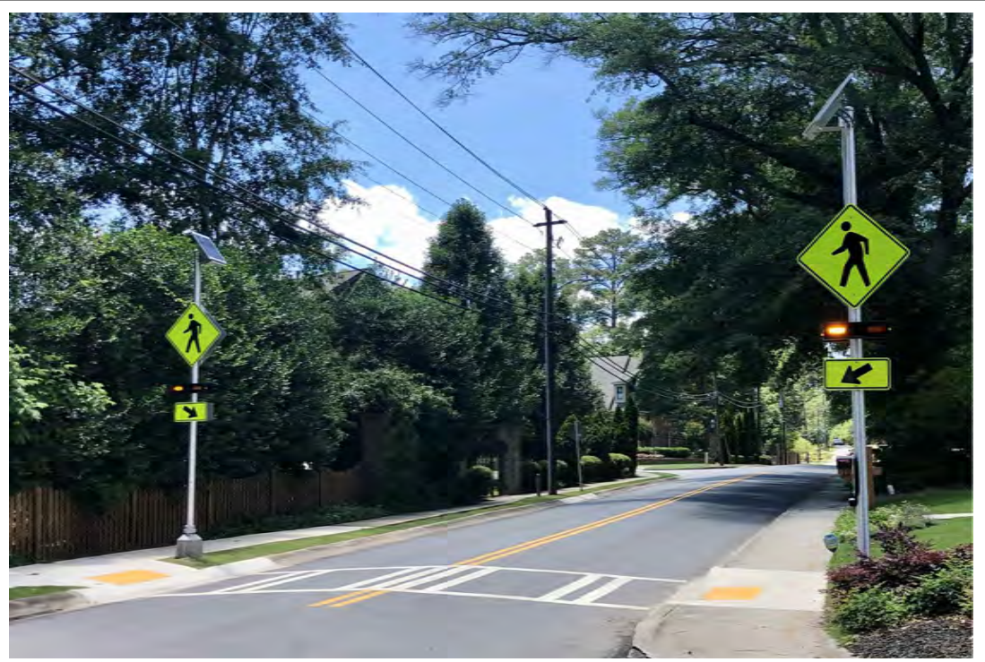
RAPID FLASHING BEACONS
